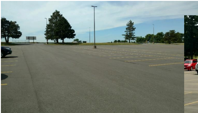
The Main Campus-E/F Parking Lot Project
