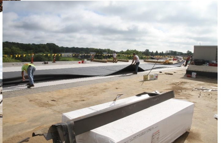
The Main Campus – Galesburg Rooftop project
