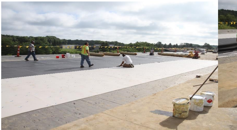
The Main Campus – Galesburg Rooftop Project
