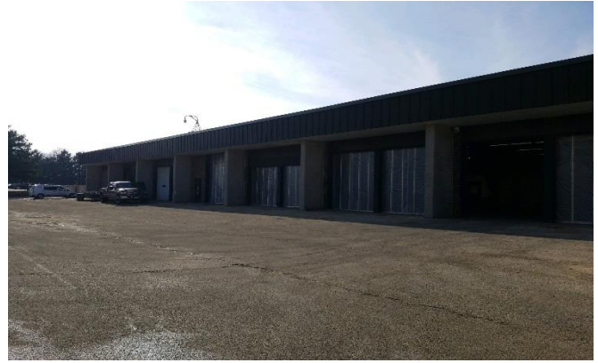
Bldg B Automotive east side of building
